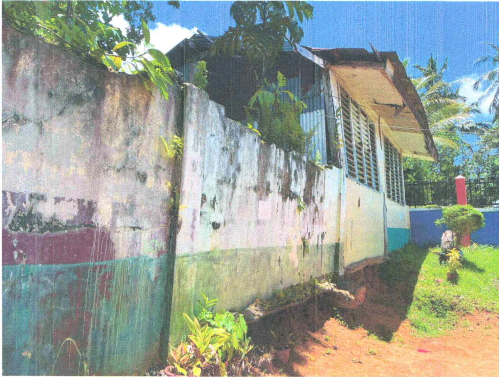
Image 3 (above): Scoured footing base due to soil erosion, buckling of wooden column due to settlement. Image 4 (below): The end wall leaned outward due to water pressure and unsupported wall to the column.
