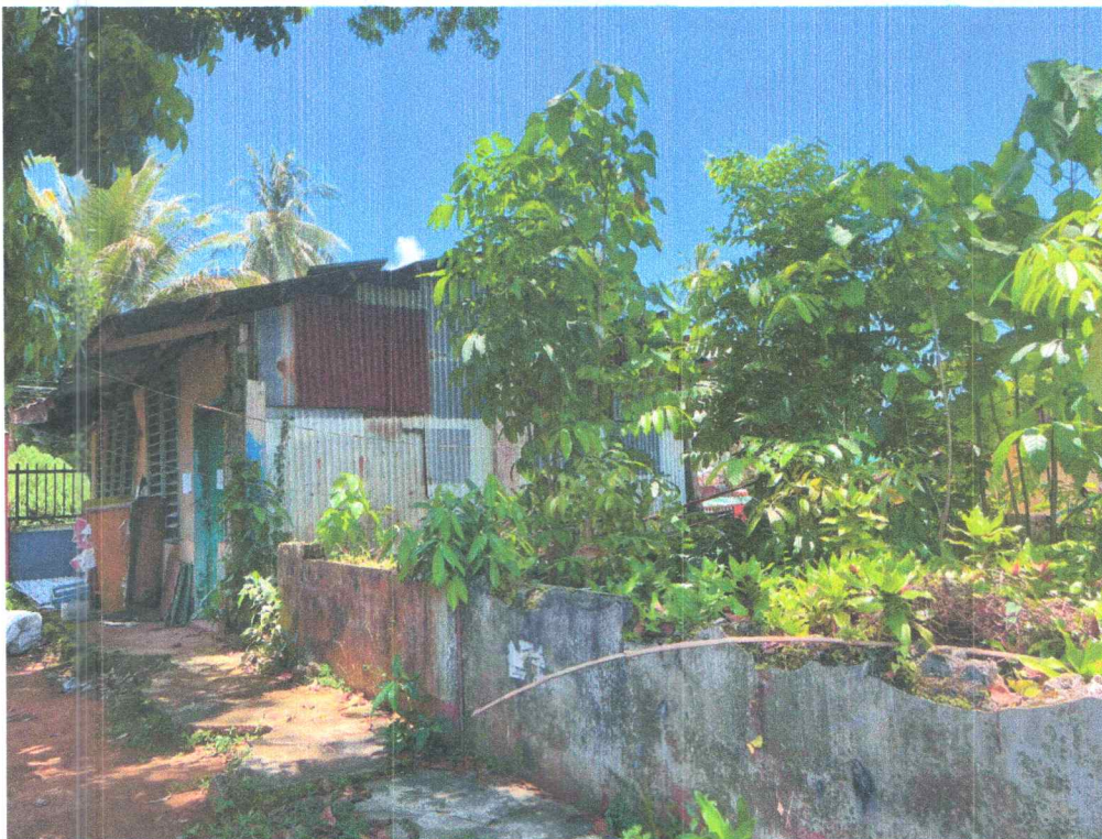
Image 1 (above): Dilapidated columns, roofing sheets, door and windows and other wooden materials. Image 2 (below): The other classroom's main structure was already demolished and replaced by vegetation growing in the area.
