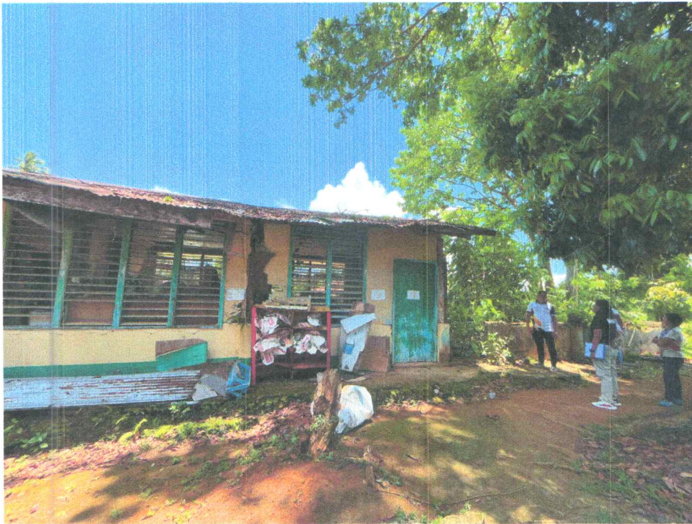
Image 1 (above): Dilapidated columns, roofing sheets, door and windows and other wooden materials. Image 2 (below): The other classroom's main structure was already demolished and replaced by vegetation growing in the area.
